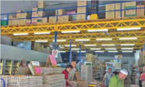
TRUSS SYSTEM MEZZANINE FLOOR
